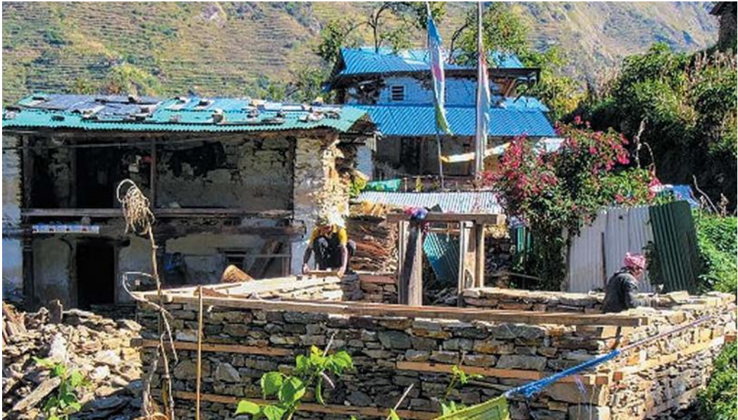
(A house under reconstruction in Tipling village, Dhading (Photo credit: Baliyo Ghar/NSET))
